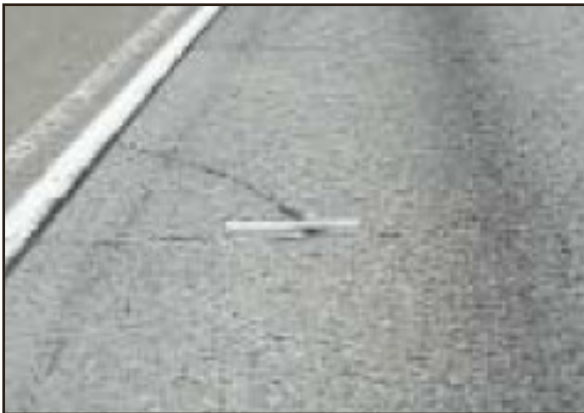
Moderate Severity Corner Break
